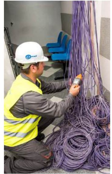
... and cables immediately before installation
