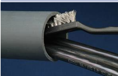
Clean duct with wire brush, solvent wipe
