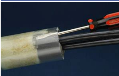
Use screwdriver to check for voids
