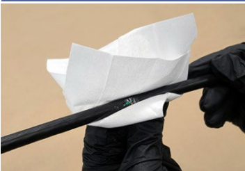
Clean area around the defect
