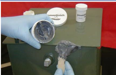
Apply PowerPatch over putty patch or leak area
