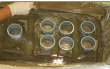
Spread the InstaGrout with a stick
