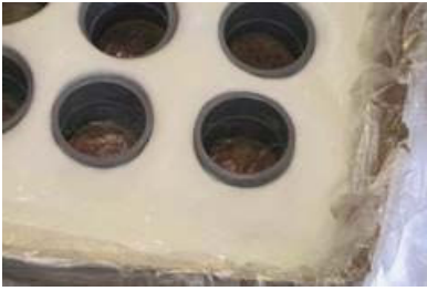
Finish installing InstaGrout
