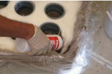
Fill in gaps with additional material
