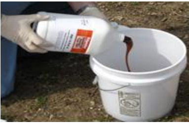
Pour 1 jug Part A, then 1 jug Part B into mixing pail
