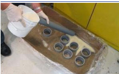
Use a 2-inch conduit to safely direct material
